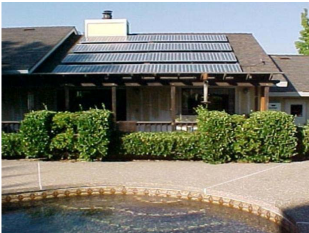
ONE OF THE SACRAMENTO MUNICIPAL UTILITY DISTRICT'S "BORROWED" SOLAR ROOFTOPS.
