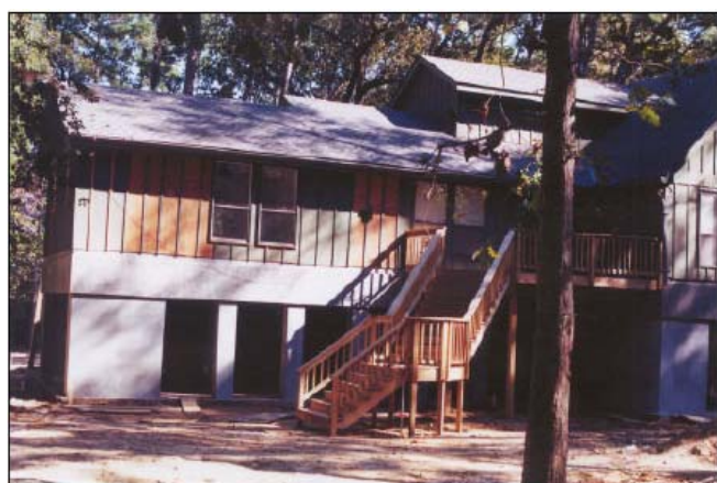
EXAMPLE OF FLOOD PROOFING THROUGH ELEVATION
