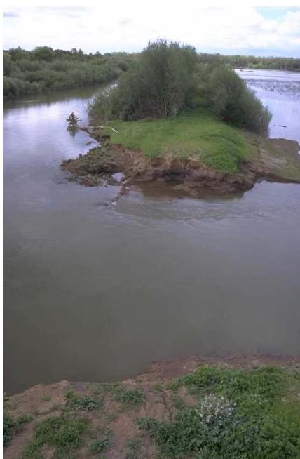
CLOSEUP OF THE LEVEE BREACH
