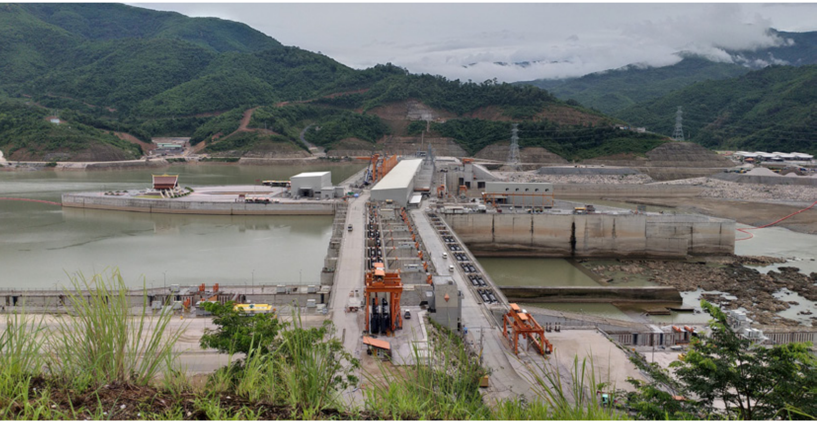
Xayaburi dam, July 2019 Photo: Thitipan Patt
