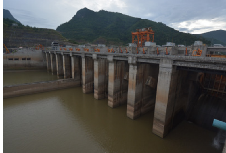
Xayaburi dam site, July 2019 / Photo: Thitipan Patt
