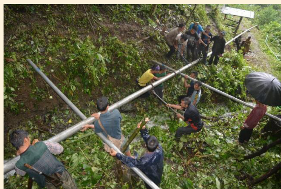
Community members installing the penstock (credit: NEPeD)
